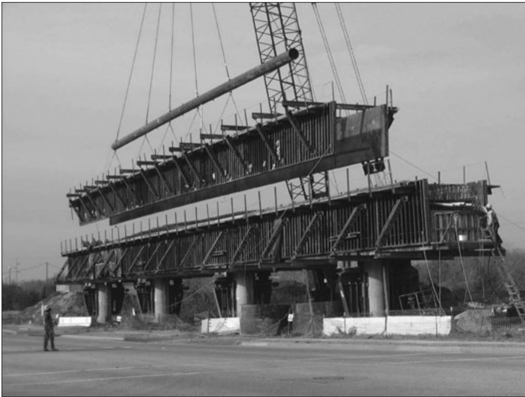
The Max-A-Form® forming system can support concrete loads over long spans without supplemental shoring. It can be used for gang-forming walls, large columns, and bridge piers. Large productivity increases over hand forming are possible, but needed workroom must be available and required hoisting equipment planned. Photo courtesy: Symons.
