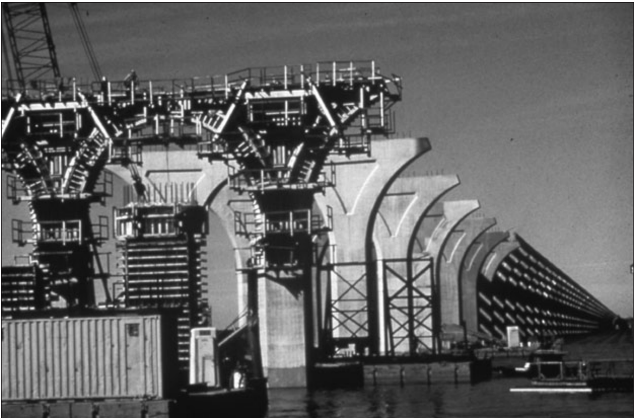
Custom-designed forms were required for these piers. The number of sets of forms purchased is a critical decision that balances the cost of the forms against increased productivity and shortened schedule that reduces general condition costs. Photo courtesy Symons.
